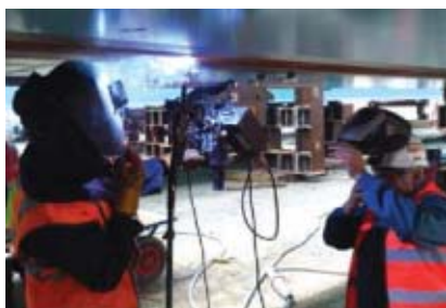
Welders observe overhead welding in the 4G position with Gulco KAT oscillator combination equipment for a bridge for the M74 motorway in Scotland.
