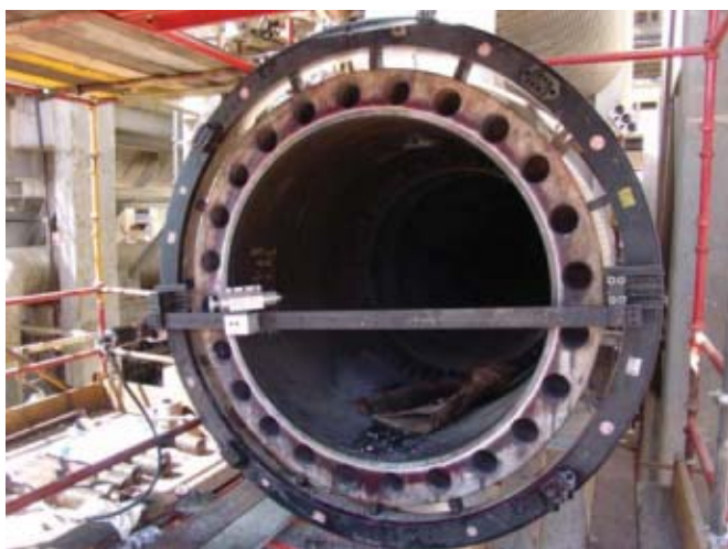
Fig. 7 — In-situ machining.
