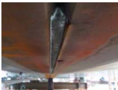
Partial joint penetration welds in butt joints for the bridge were completed in one run for passes one and two.
