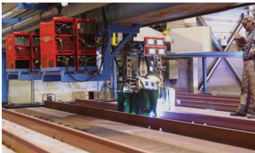
Fig. 3 — Automation is used to join both sides of the reinforcement plate to the floor area using the tandem wire welding system.
