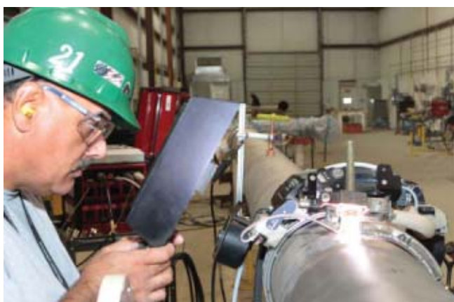
Fig. 4 — A welding operator viewing the progress of an orbital weld on titanium pipe.
