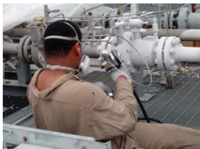
Fig. 8 — Combustion wire spraying a pressure gauge with aluminum, 300 \mu m (12 mil).
