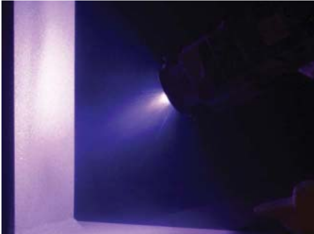
Fig. 2 — Close-up shot of an arc spray system placing 85/15 (zinc/aluminum) onto a dam gate.
