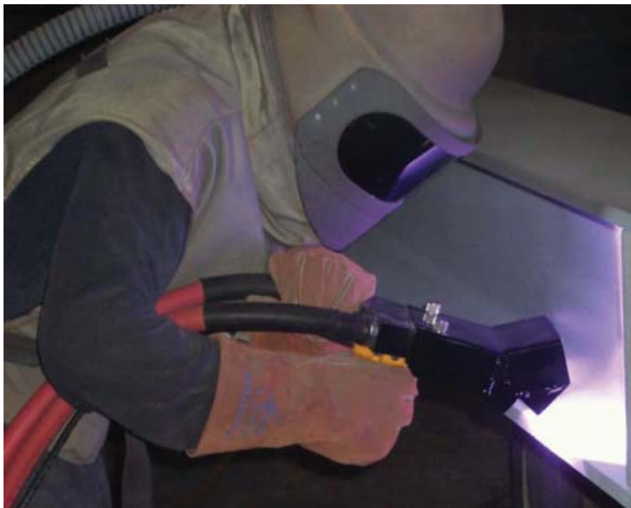
Fig. 1 — An operator uses the arc spray system for applying zinc wire onto a support beam.
