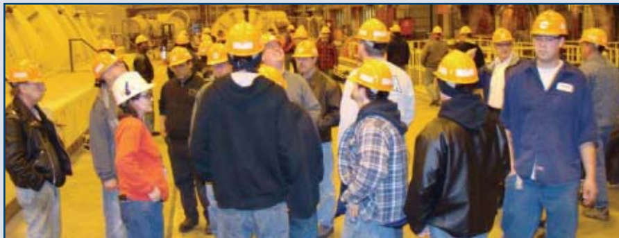
Racine-Kenosha Section members toured the Wisconsin Energy P-4 power plant in April.
