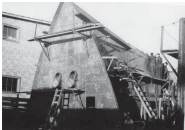
Fig. 3 — This upended bow section of a destroyer escort was completed on the ground before erection.
