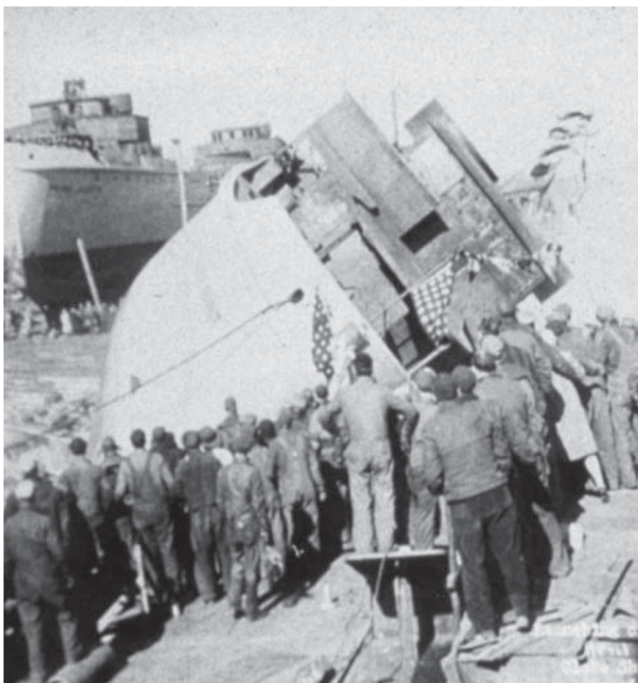
Fig. 2 — As more ships were launched in the Globe yard, more of the superstructure of each ship was added before launching, making the vessels increasingly top heavy. This one almost rolled over during launching. From then on, the engines were installed before launching to lower the center of gravity.
