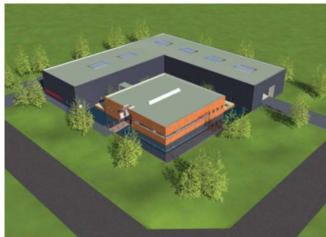
An architectural rendering of the Magnatech facility under construction in The Netherlands.
