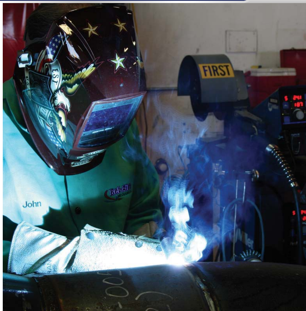
Fig. 2 — The new technology yields uniform high-quality welds at twice the former productivity using operators with a wide range of skill levels.
