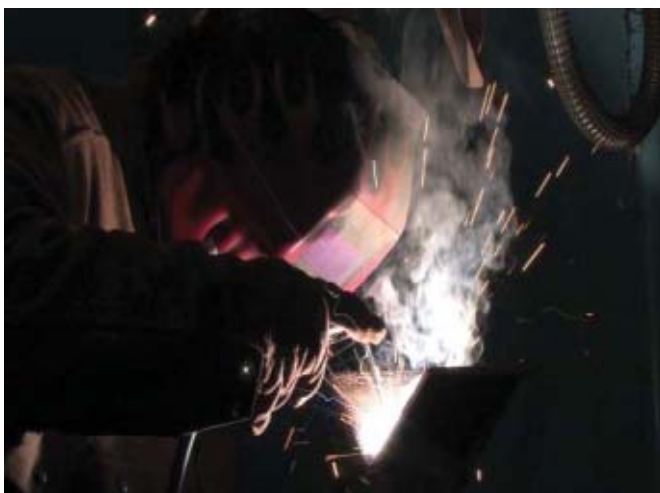
The Rankin Career & Technical Building of Hinds Community College in Pearl, Miss., officially opened recently. Coby Gaines, an attendee of night classes, uses shielded metal arc welding with a 1/8-in. 7018 electrode to perform a fillet weld on an inside corner joint in the 1F position. (Photo courtesy of Barin von Foregger/Hinds Community College.)
