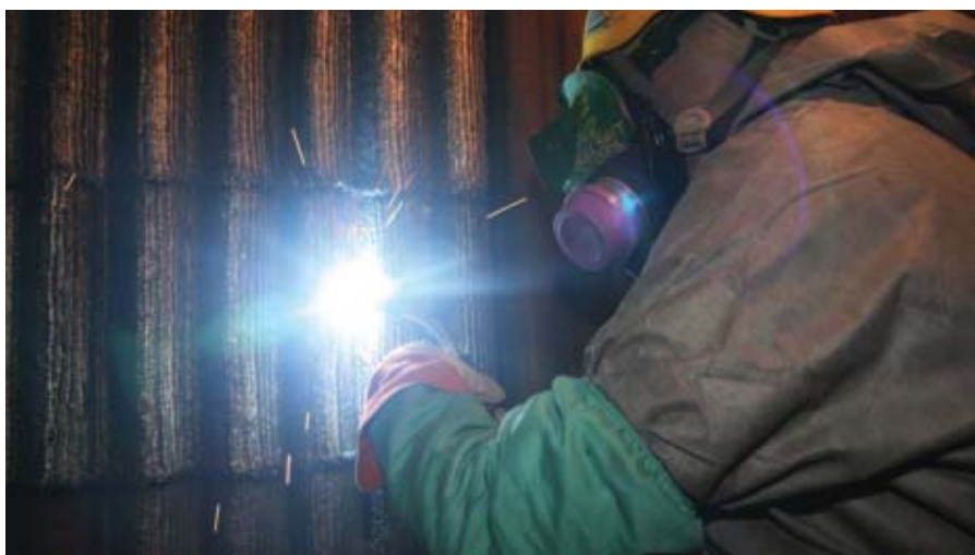
Fig. 4 — Operators need to be able to hold a short arc length for maximum weld pool control.
